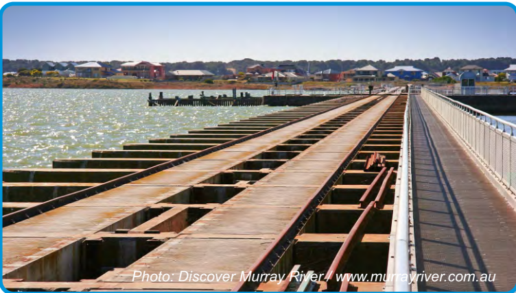
Left: 1 of 5 of the Goolwa Barrages built to stop salt water intrusion in the lower Murray River.
