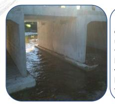
Box culverts can open up access to upstream habitat as they have better light levels, lower velocities and are blocked less by debris than pipe culverts.
