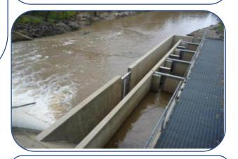
Vertical-slot fishways assist fish passage through barriers up to 6m high. (Photo: Catchment Solutions)
