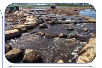
Rock-ramp fishways are the most common remediation for barriers to 2m high. They consist of a series of resting pools that help the fish make their way upstream and downstream and are designed to function at low flows. (Photo:
