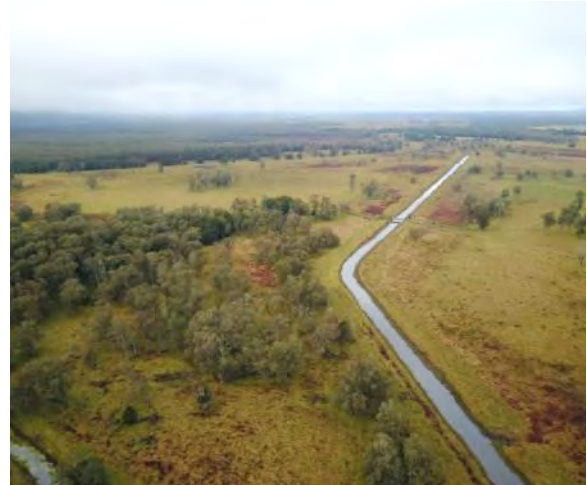
22: Tucki Canal looking downstream
