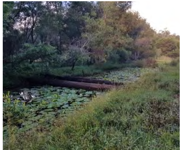
12: Significant blockages of Stony Island Drain
