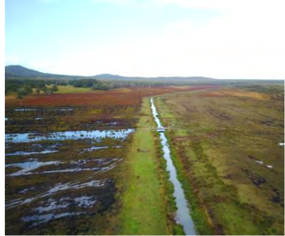
20: Looking downstream along Slatteries Drain
