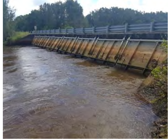
2: Downstream Bagotville Barrage flowing out
