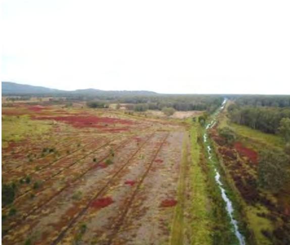
21: Hendersons Drain, looking downstream.
