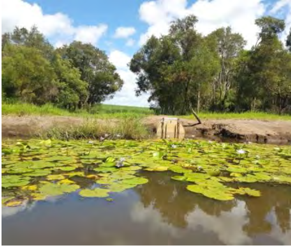
7: Typical minor drain floodgate, Stibbards Creek
