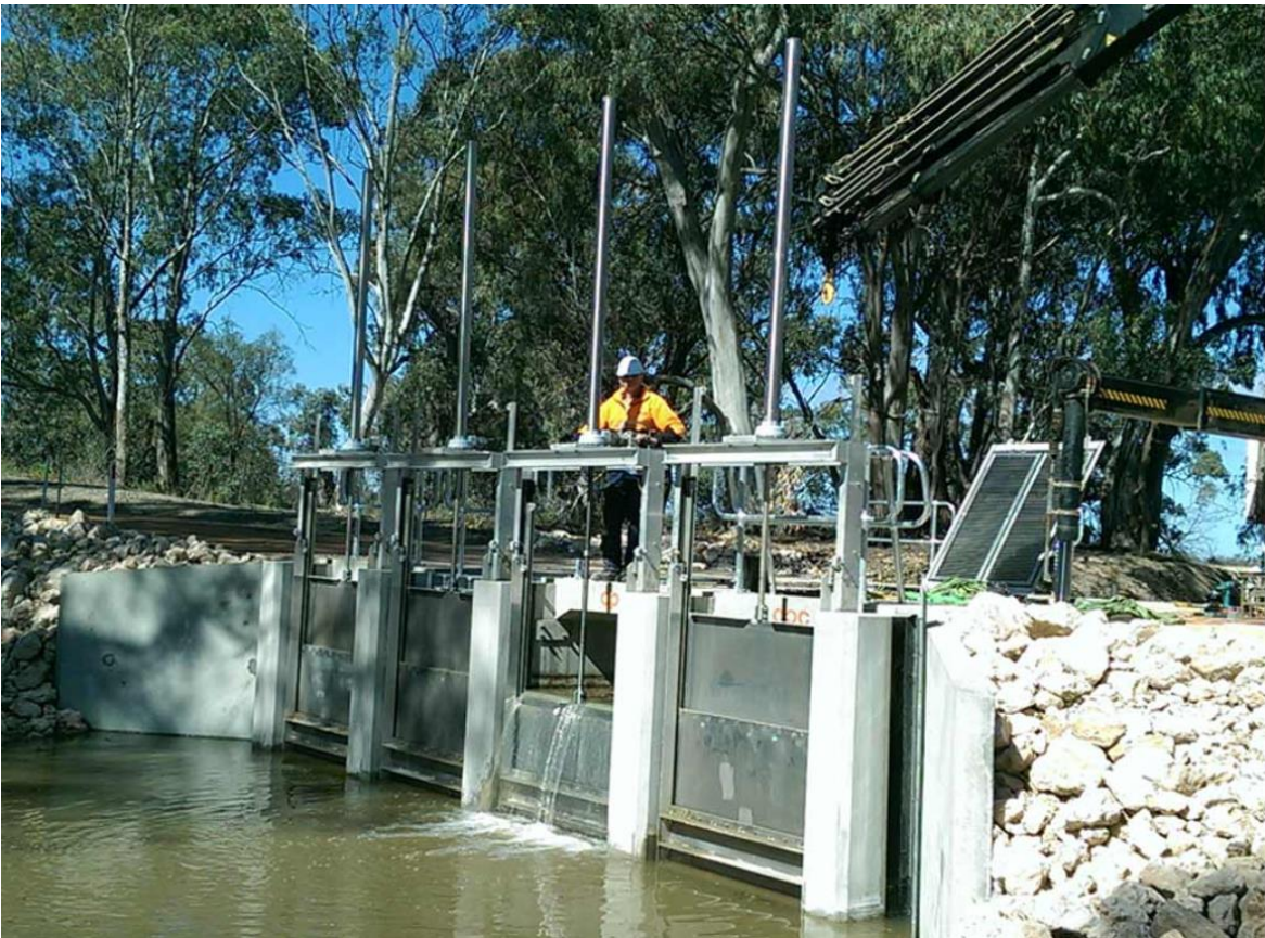
Figure 3.3 Multi-leaf gates operating (AWMA, 2022a)
