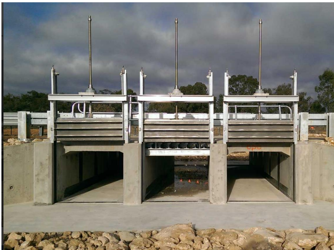
Figure 3.2 Multi-leaf gates fully open (AWMA, 2022a)
