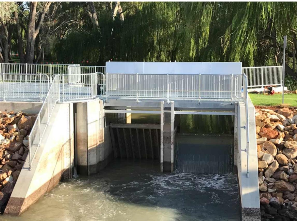
Figure 3.4 Lay flat gate (AWMA, 2022c)
