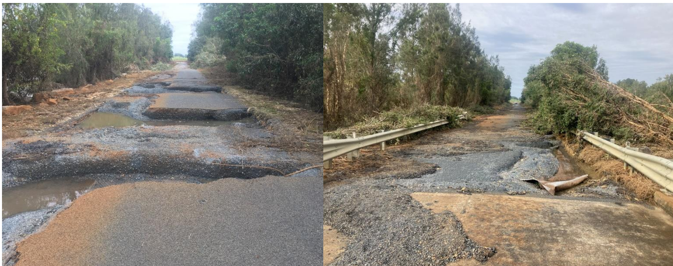
Figure 2.9 Post flood damage to Old Bagotville Road at the barrage
