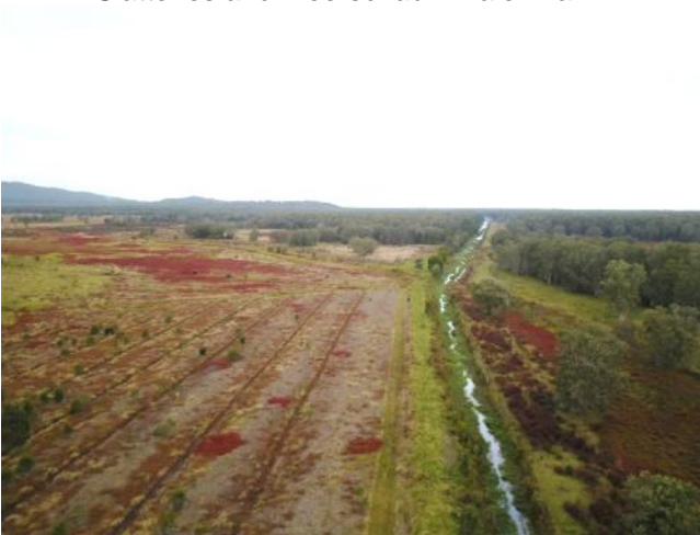
21: Hendersons Drain, looking downstream.
