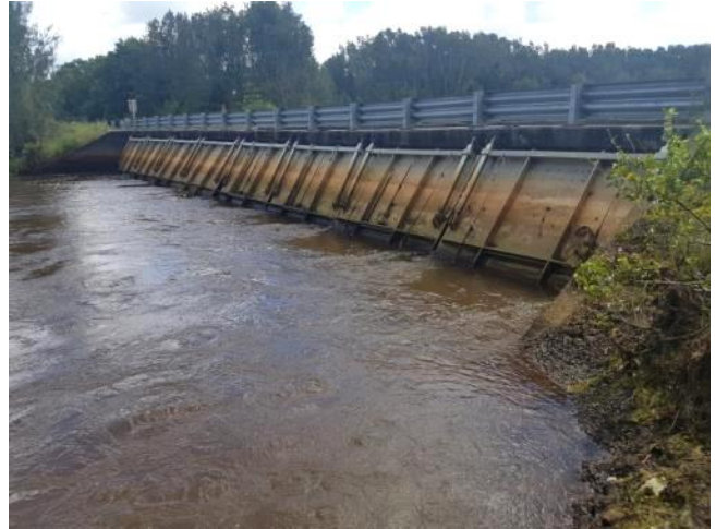
2: Downstream Baggotville Barrage flowing out
