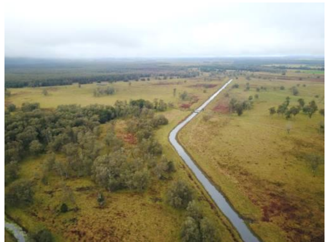
22: Tucki Canal looking downstream (Nature Reserve Drain visible in the bottom left)
