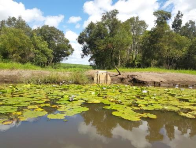
7: Typical minor drain floodgate, Stibbards Creek
